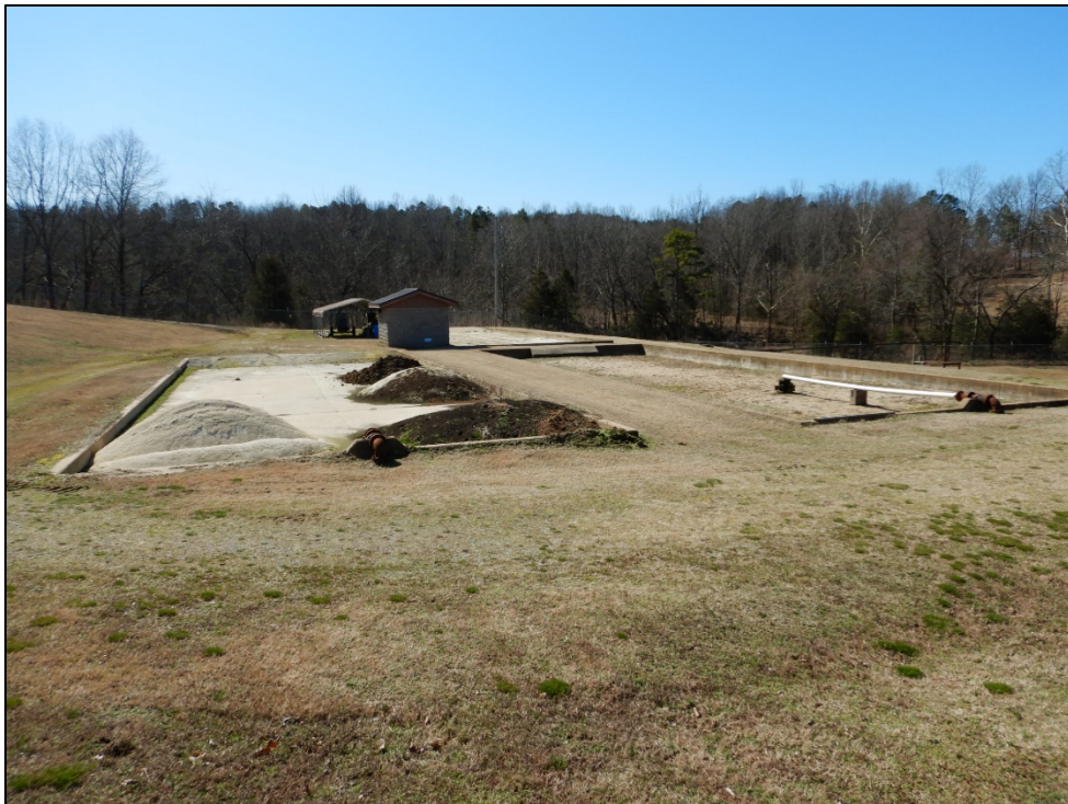
Photograph 12. Sludge drying beds and staging bed.
