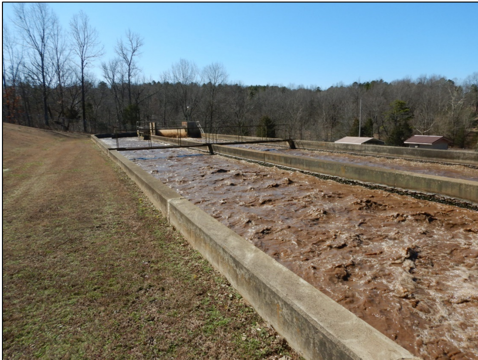
Photograph 2. Oxidation ditch.
