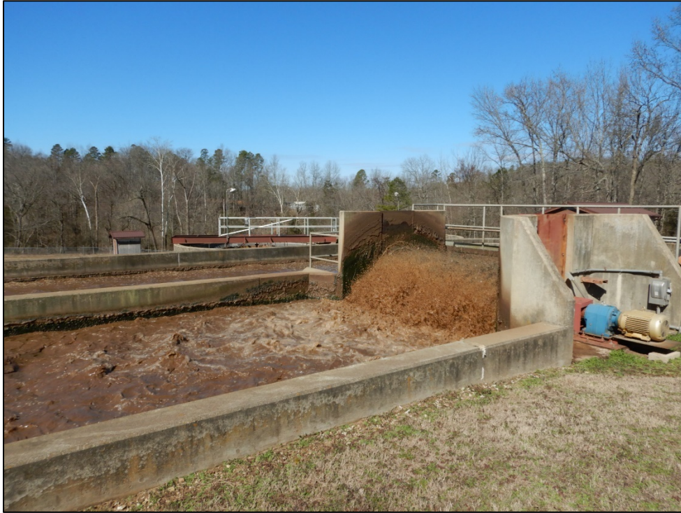
Photograph 3. Oxidation ditch.
